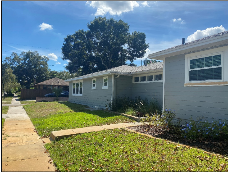
Figure 4: Staff photograph of east elevation of property, facing southwest from 32 nd St. N.
